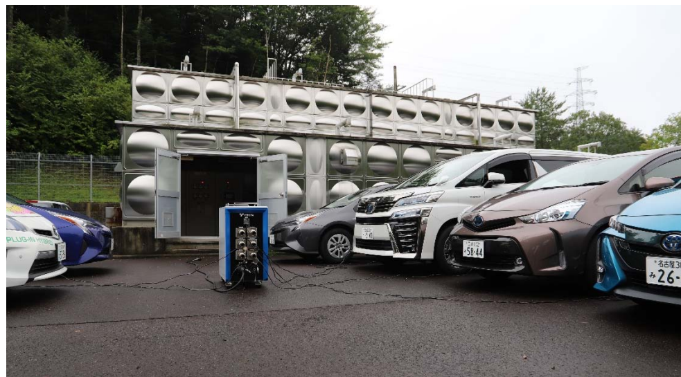
Feasibility test for operating water distribution pump
